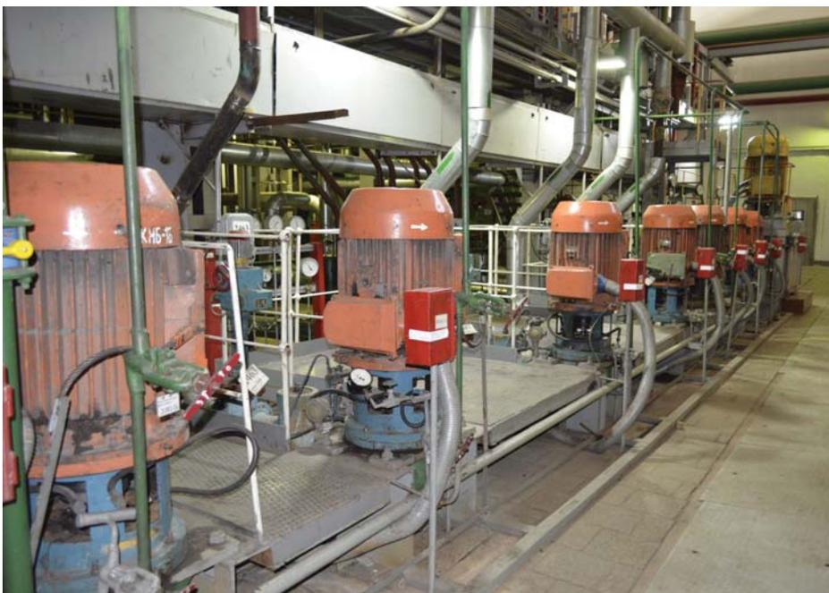
*Group of condensate pumps, KsV 125-140 series, made by HMS Group for PT 80-140 turbine, have recently undergone the upgrade.*
