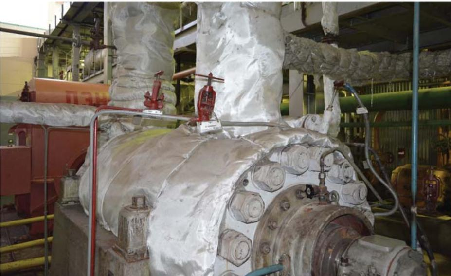
*Feed water barrel pump, PE 580-185 -5 series made by HMS Group, in glass wool insulation.*
