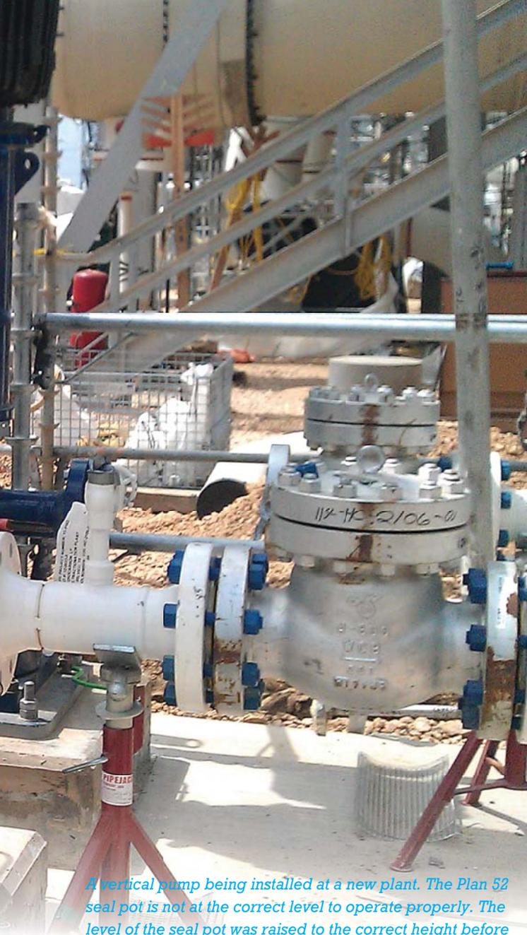
*A vertical pump being installed at a new plant. The Plan 52 seal pot is not at the correct level to operate properly. The level of the seal pot was raised to the correct height before the installation was complete.*
