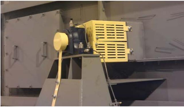
*This picture shows a pillow block bearing with accelerometers installed for continuous vibration monitoring on a new installation.*
