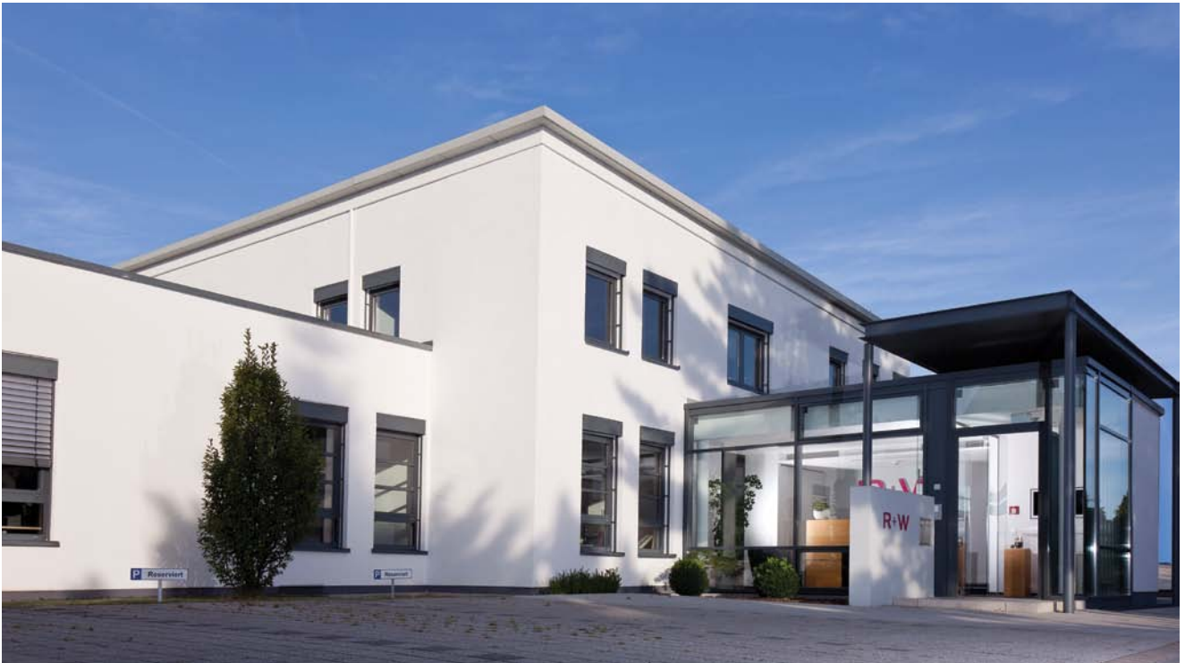
R+W Antriebsysteme GmbH headquarters in Klingenberg am Main, Germany.
