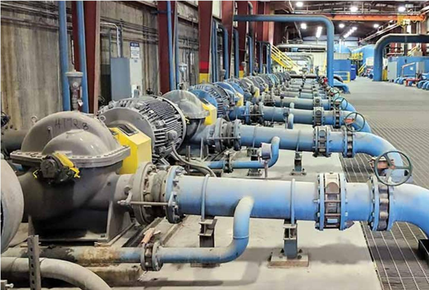
*Pumping operation with expansion joints in a steel mill.*
