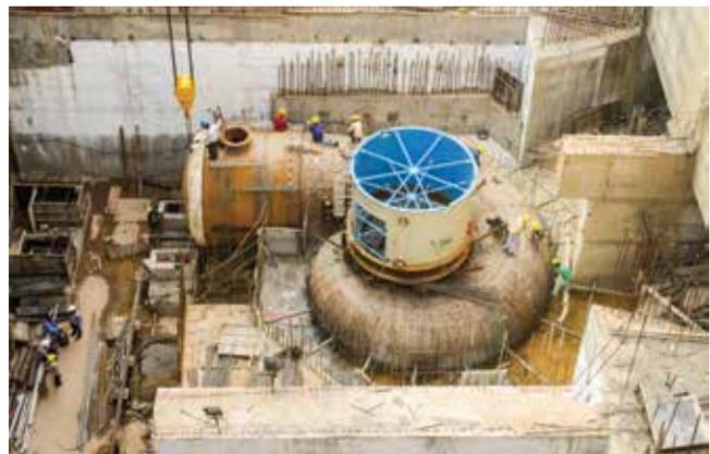
A recent project required a multi-stage lift irrigation system in the Indian state Telangana. ANDRITZ supplied 25 vertical volute pumps for three pumping stations, each with an efficiency of up to 90%.
